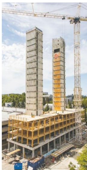
Figure 3 Construction method ((CWC), 2017)
